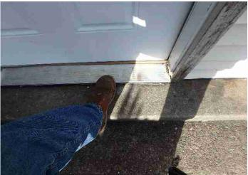
13.11 - Recommend consulting a door contractor or equal to cap all exposed wood around the rear exterior door of this home. There are spaces between the rear door jamb and the siding that will allow water to migrate between the building materials. There are exposed pieces of wood that should be capped or painted to protect them from the weather.
